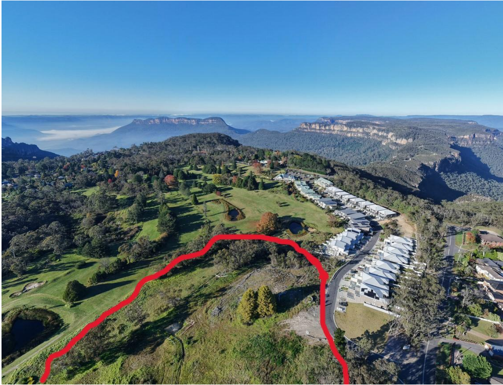
Figure 5.1: Proposed development site outlined in red, showing potential impact on views from the adjoining Planetary Health Precinct (old golf course) and adjoining properties.
