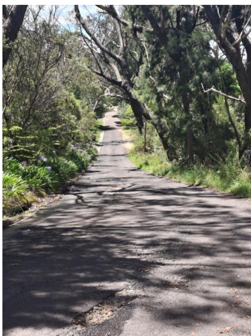
Figure 6.1 Glencoe Rd looking north (E Howard)
