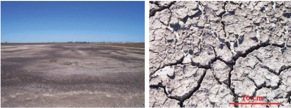
FIGURE 4. Evaporation ponds at Dalby (QLD) showing evidence of cracking. 101
