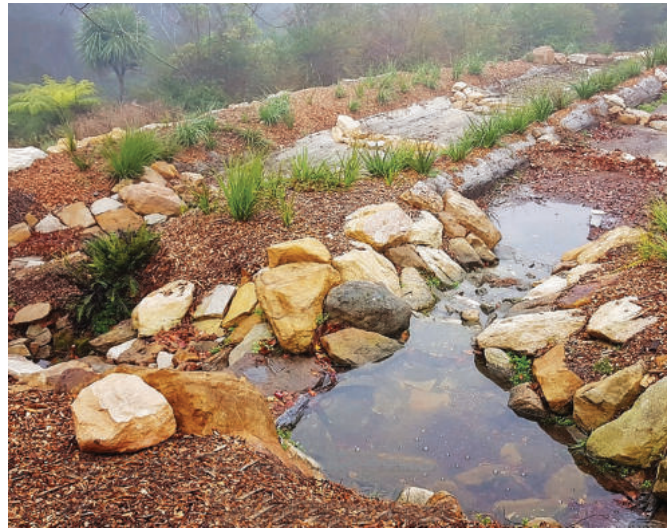
A stormwater biofiltration system improving water quality at Leura Falls Creek.
