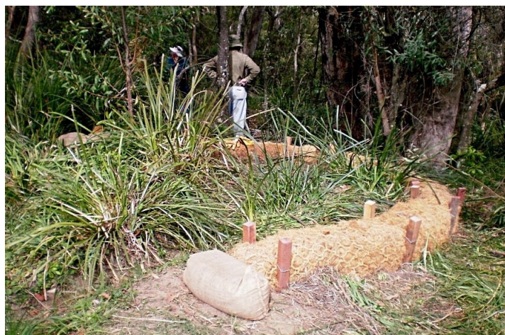
Soft coir logs minimise stormwater and weed seed flows into healthy bushland (P Ardill)
